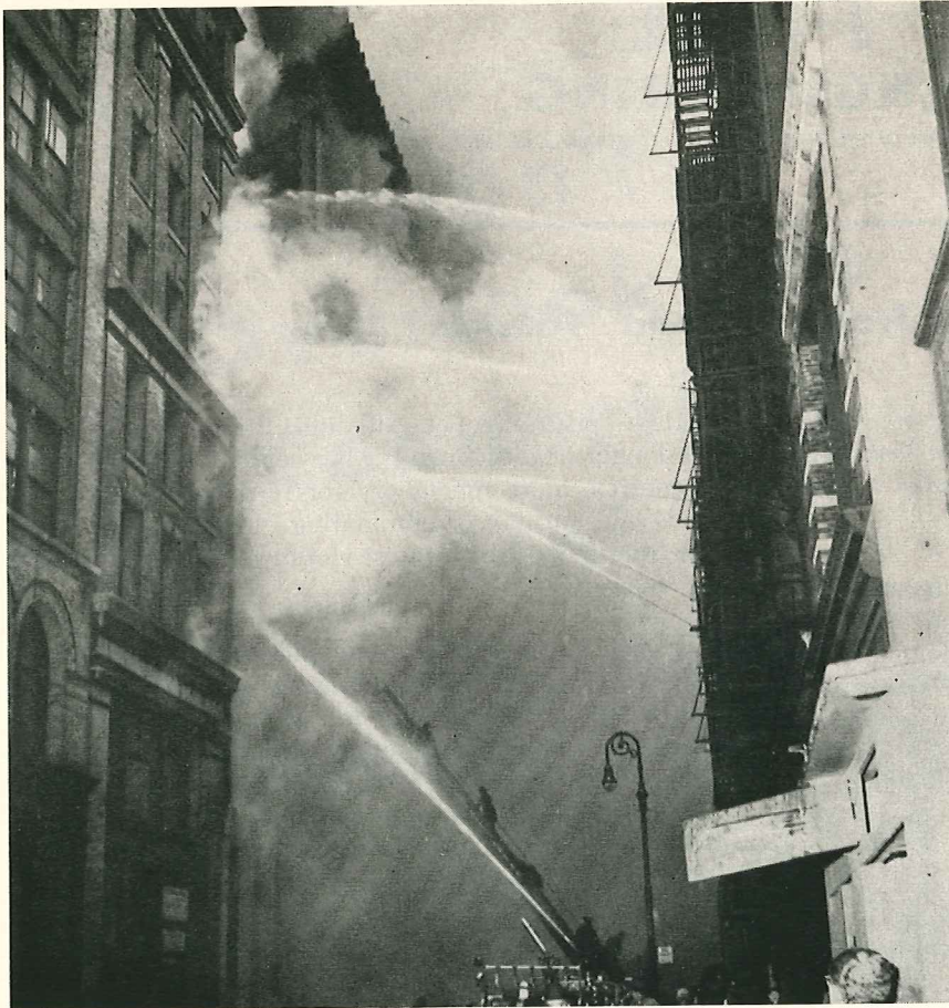
Heavy streams are directed into burning loft building from every vantage point in the rear (Mercer Street). Extreme depth of structure limited penetration. Men of Ladder 20 are shown
