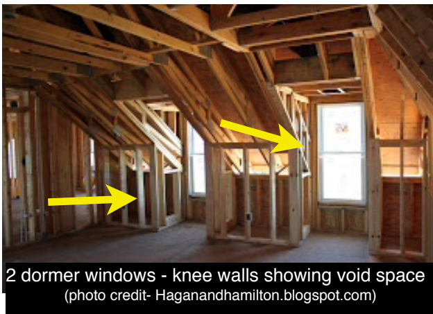
Use the window sill as a guide from outside to vent knee walls- relieves heat on interior crew (photo credit- westerninsulation.ie)
