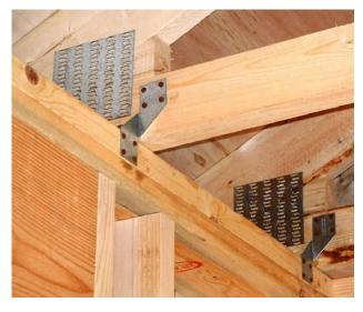
Photo 1 shows a common method used to reinforce the connection between a rafter or roof truss and the double top plate of a woodframe wall. It shows a lightweight metal strap or clip (to the right of the manufactured gusset plate) attached with nails in addition to the number of nails required by code or architect to attach the roof truss. Note that for this hurricane tie to be effective, the proper number and size of nails must be used: every hole in the tie must have a nail into wood.
